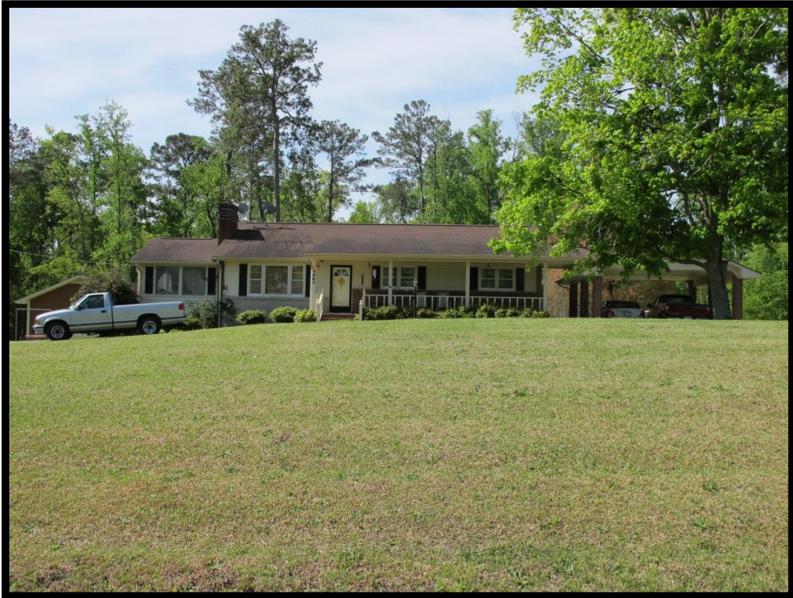
Figure 57: House (B), Looking South.
