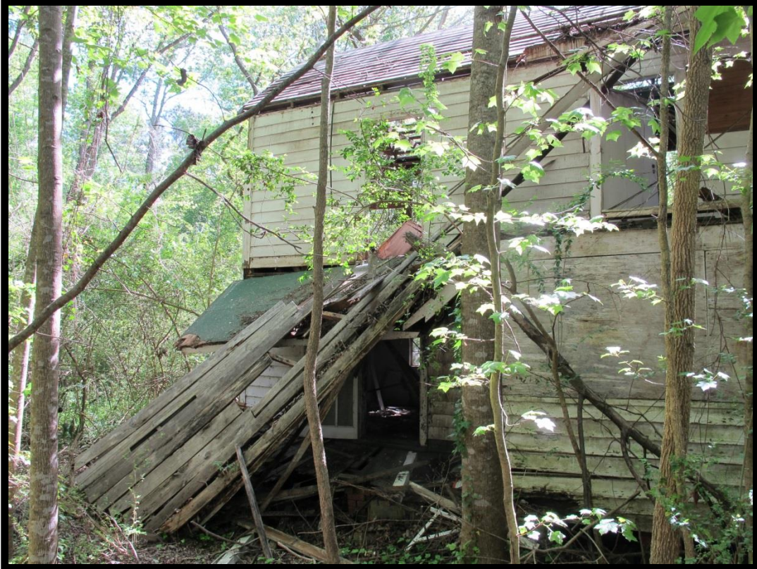
Figure 50: Reel House (PM0256), Rear Wing, Looking Northeast.
