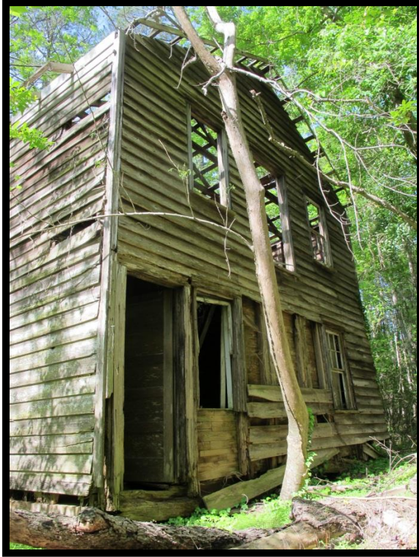
Figure 51: Reel Store (PM0256), Rear Gable End, Looking Southwest.
