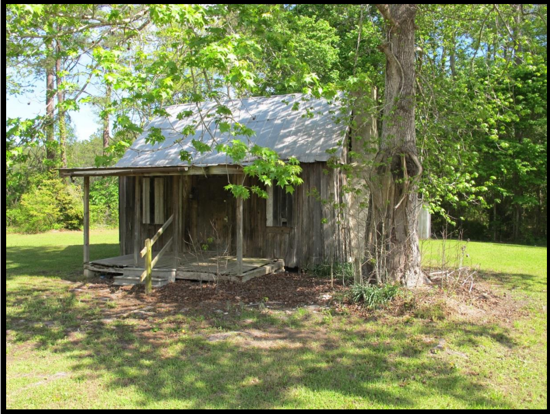
Figure 5: Alex Brinson House (# 1), Looking Northwest.
