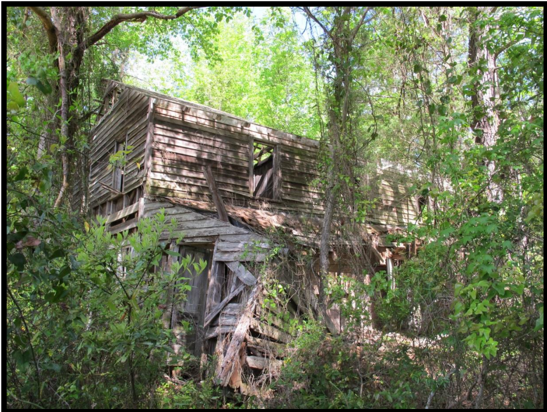
Figure 48: Reel Store (PM0256), Looking Northwest.
