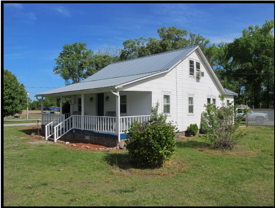
Figure 40: Benjamin Brinson House (PM0254), Looking Northwest.
