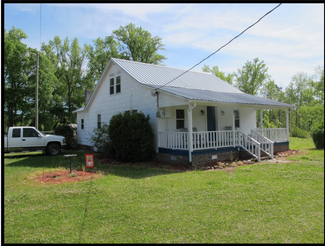
Figure 39: Benjamin Brinson House (PM0254), Looking Northeast.
