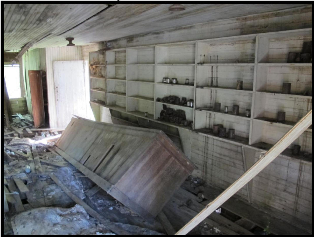
Figure 52: Reel Store (PM0256), Interior, Looking Northeast.
