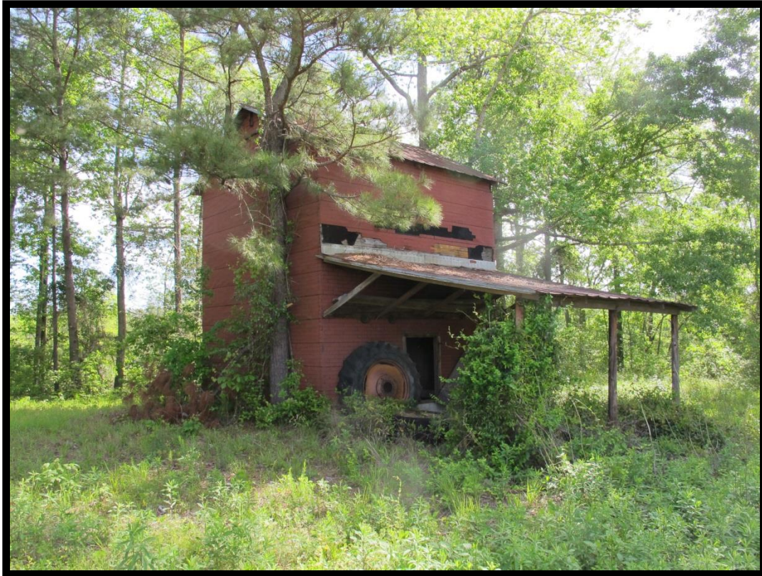
Figure 45: Benjamin Brinson House (PM0254), Tobacco Barn, Looking Northeast.
