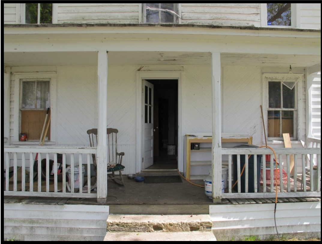
Figure 26: Levin Paul House (# 3), View of Sheathing on Southwest (front) Elevation.
