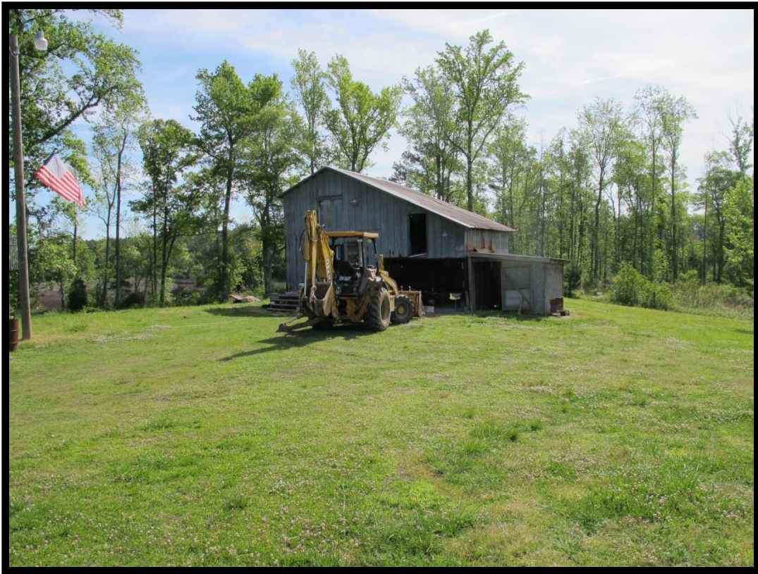
Figure 43: Benjamin Brinson House (PM0254), Pack House, Looking Northeast.
