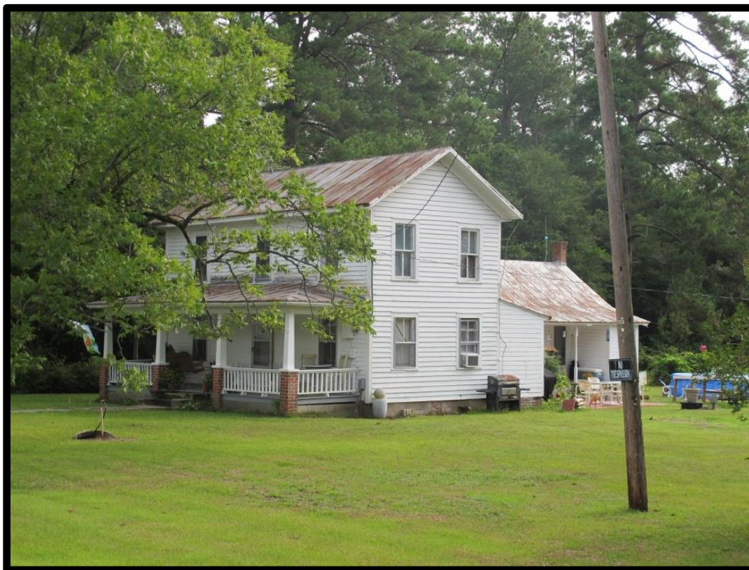
Figure 35: Hunnings House, 1494 NC 306, Looking Northeast.
