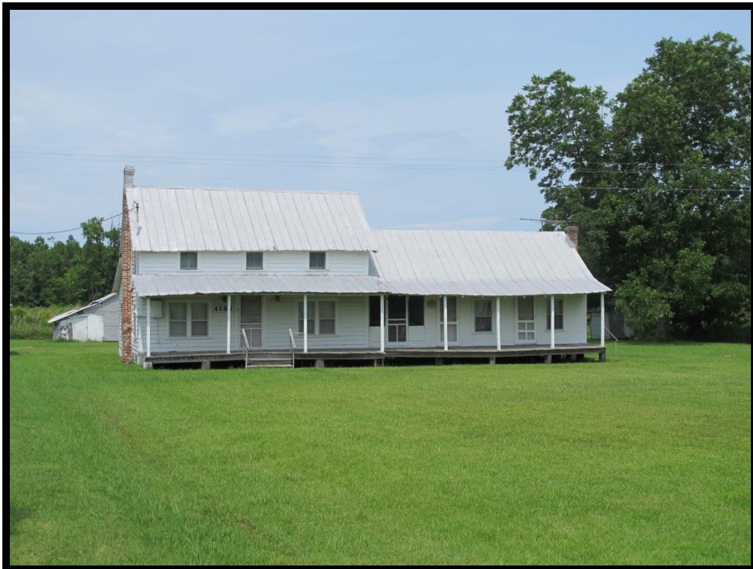
Figure 21: Buell T. Potter House (PM0419), Looking Northeast.
