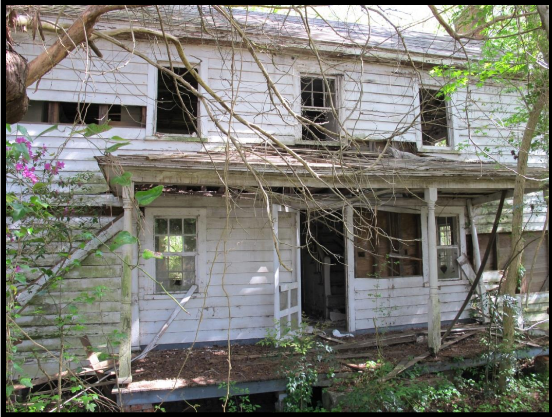
Figure 49: Reel House (PM0256), Front Elevation, Looking Northeast.
