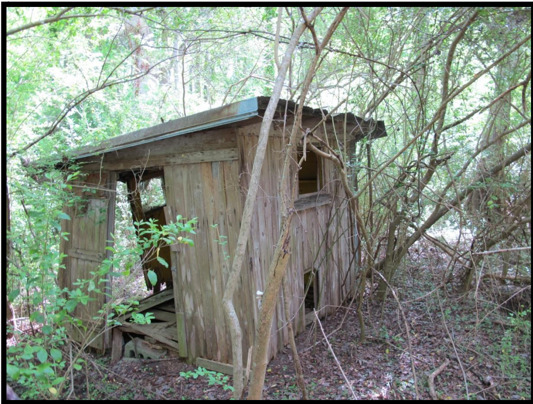
Figure 54: Reel House and Store (PM0256), Chicken Coop, Looking Northeast.
