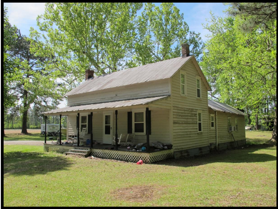
Figure 15: George R. Brinson House (# 2), Looking Southeast.
