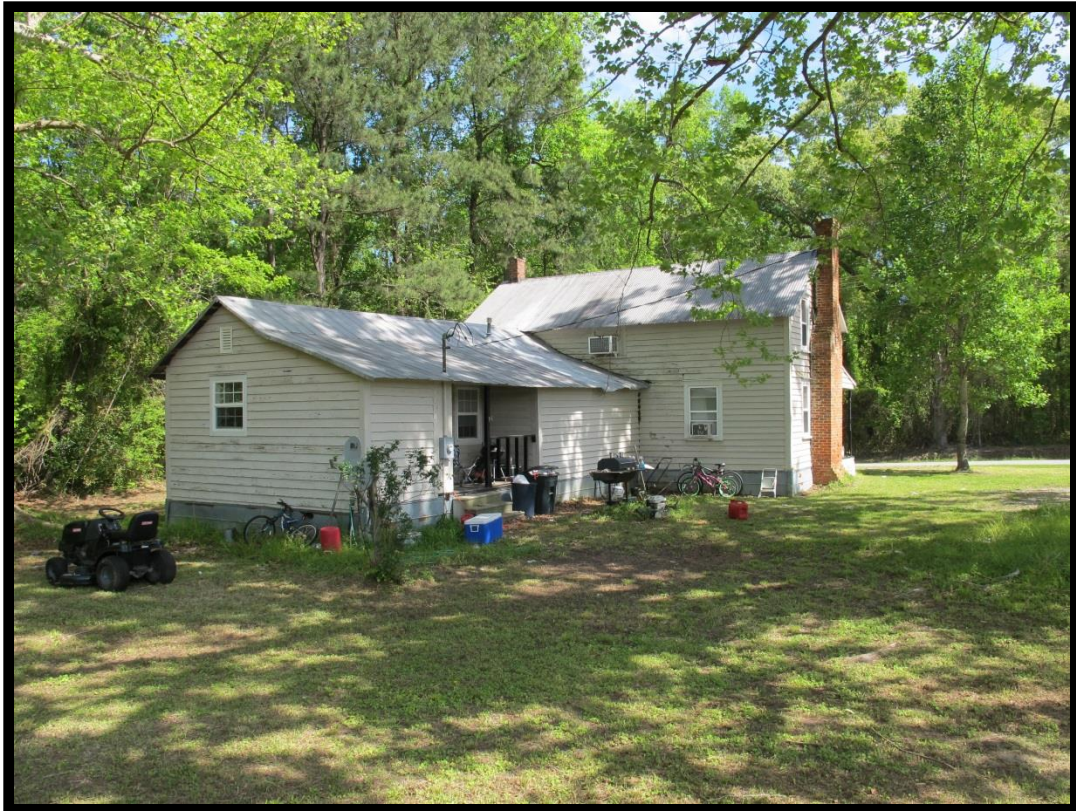
Figure 16: George R. Brinson House (# 2), Looking Northwest.
