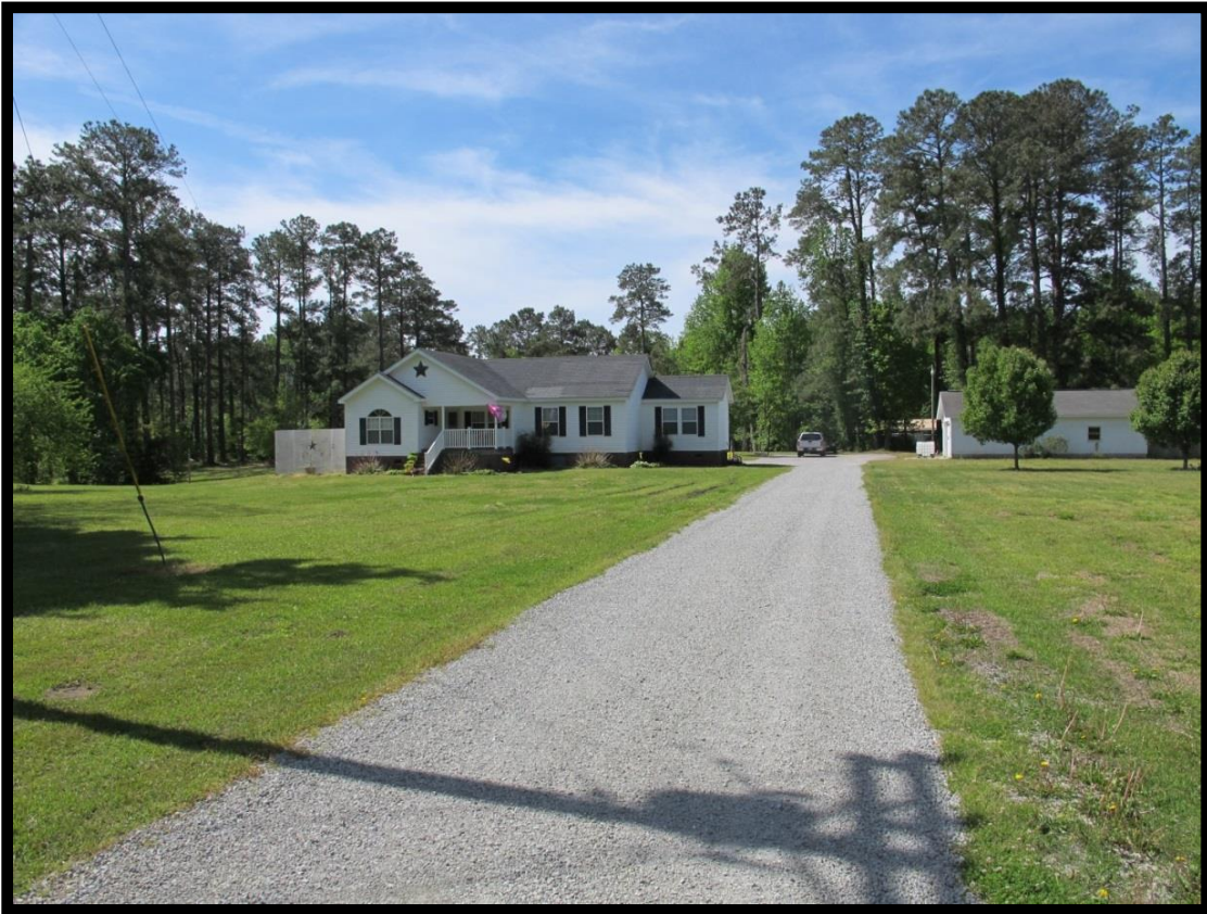
Figure 59: House (E), Looking Southwest.
