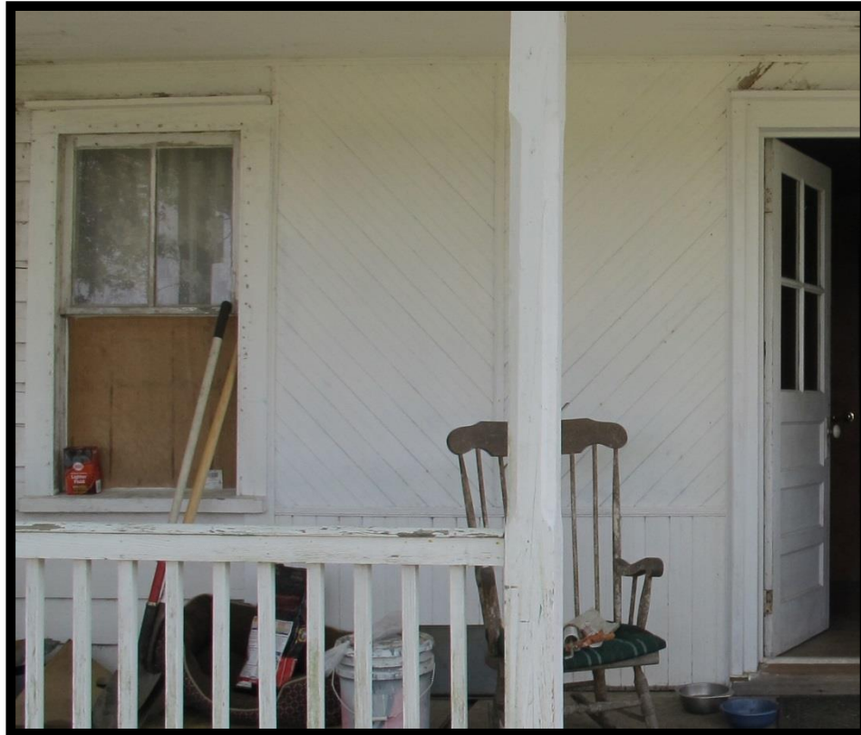
Figure 27: Levin Paul House (# 3), Detail of Sheathing on Southwest (front) Elevation.
